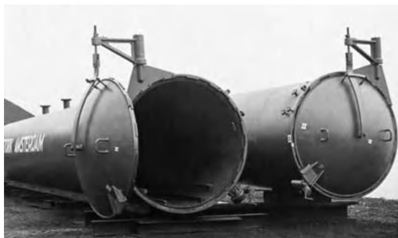
Plate 13.2 Horizontal bunch sterilisers with bayonet-type doors. (Gebr. Stork & Co.)
