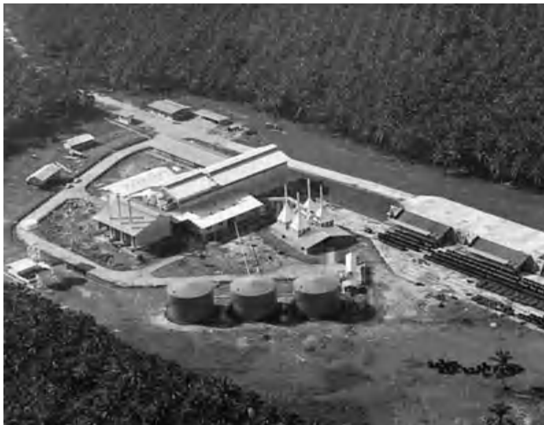
Plate 13.1 A large mill of 60 tonnes per hour capacity serving 8000 hectares in Malaysia.
